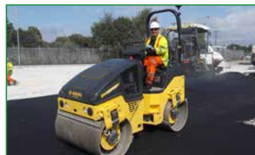
All driveways are compacted using this
